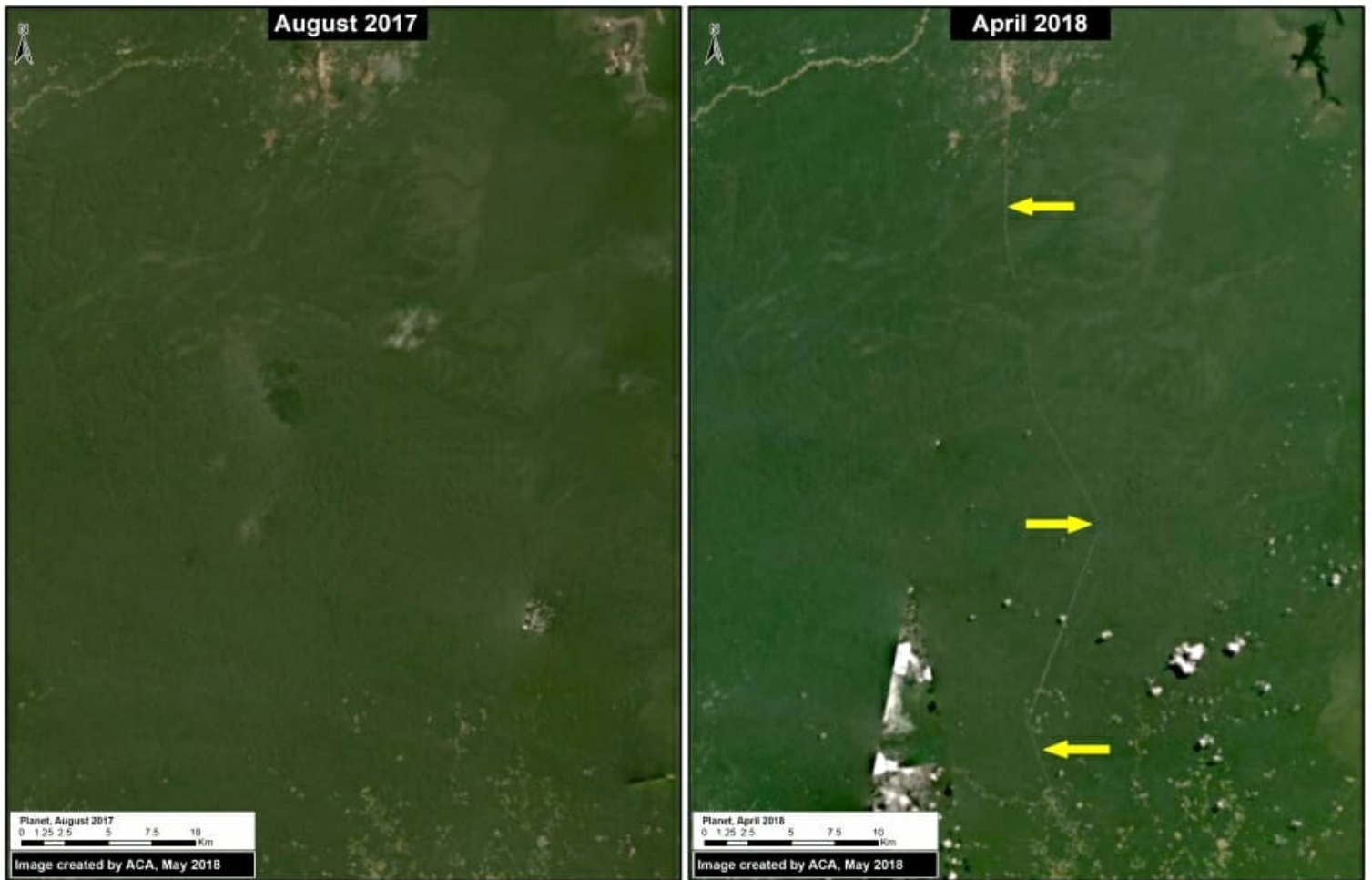
Image C. Road construction. Data: Planet.
